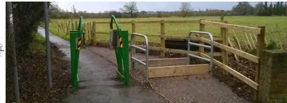
fig 3-44 Example of how NMU route can be designed to accommodate occasional maintenance access
